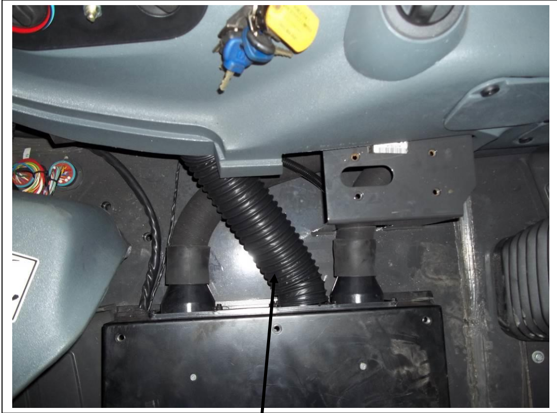
Flex hose connected to the evaporator box going to the additional louver. May exist in newer models.
